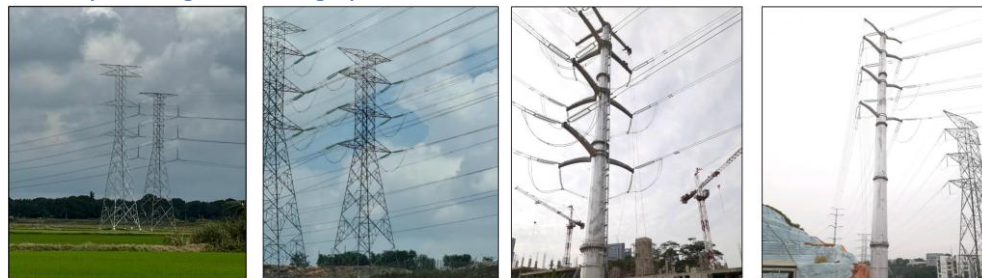
Figure 3: Examples of lattice pylon towers (two images on the left) and monopole pylon towers (two images on the right).
