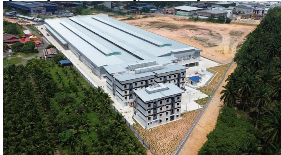
Figure 17: Progress of new manufacturing plant as at mid-Aug 2025
