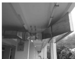
Installation of ventilation fan system for a high rise residential property in Selangor
