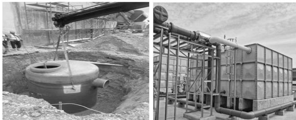
Figure 6: Value-added Components Featuring Oil Separator (left) and Rainwater Harvesting System (Right)
