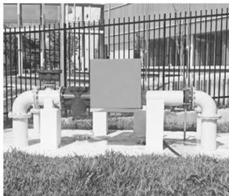
Figure 5: Construction and Installation of Piping Systems Featuring Metering Point (left) and Cold and Hot Water Systems (Right)
