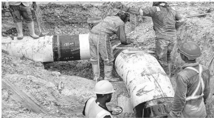
Figure 8: Trenching and Installing Water Supply Infrastructure Piping
