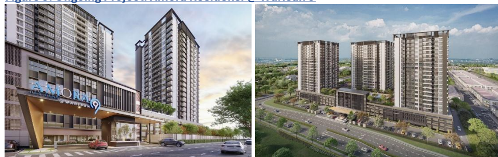
Figure 9: Ongoing Project: Amora Residensi @ Warisan 9
