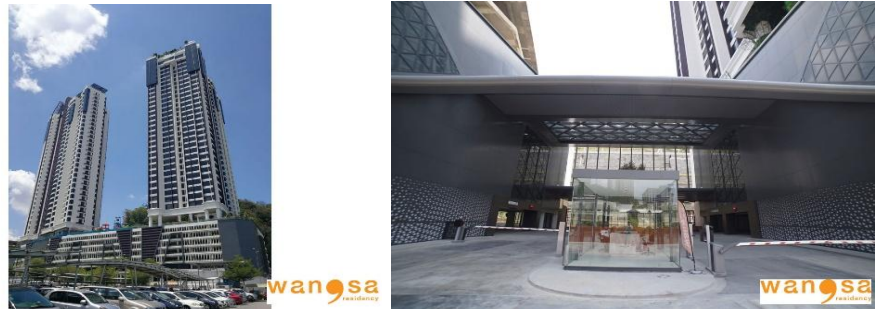
Figure 10: Ongoing Project: Wangsa 9 Residensi (Wangsa Maju, KL)
